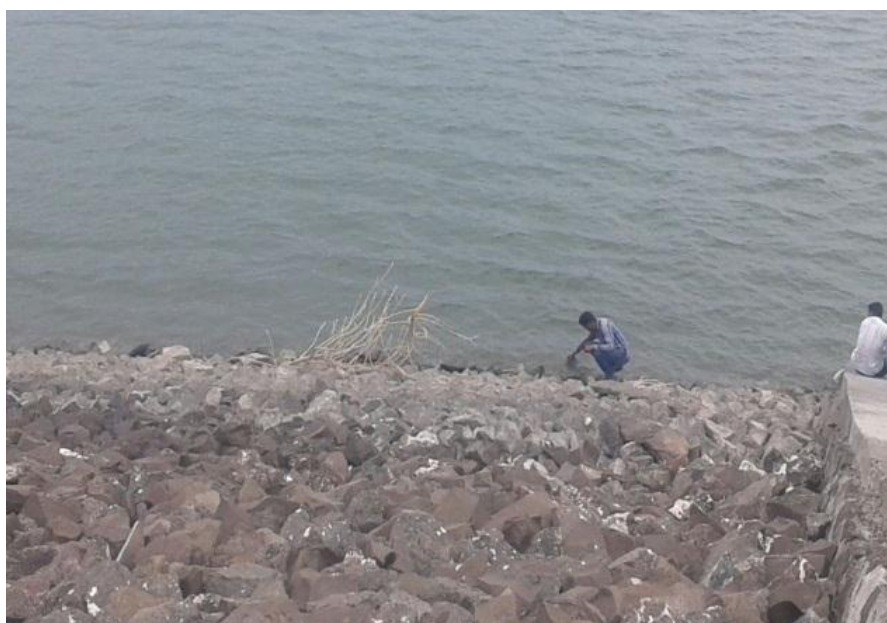
Figure 2. Study location: Aadhala -1 (Spot -1). River in Devthan Village in Akole Taluka of Ahmednagar district of Maharashtra state, India.
